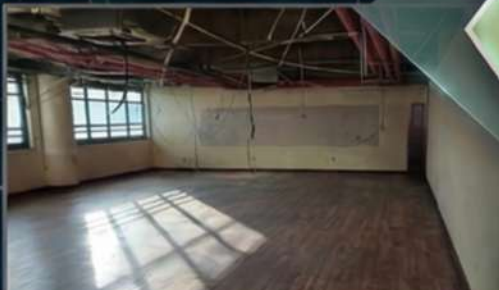
[BEFORE-공사중 OUTDATED SHELL]
